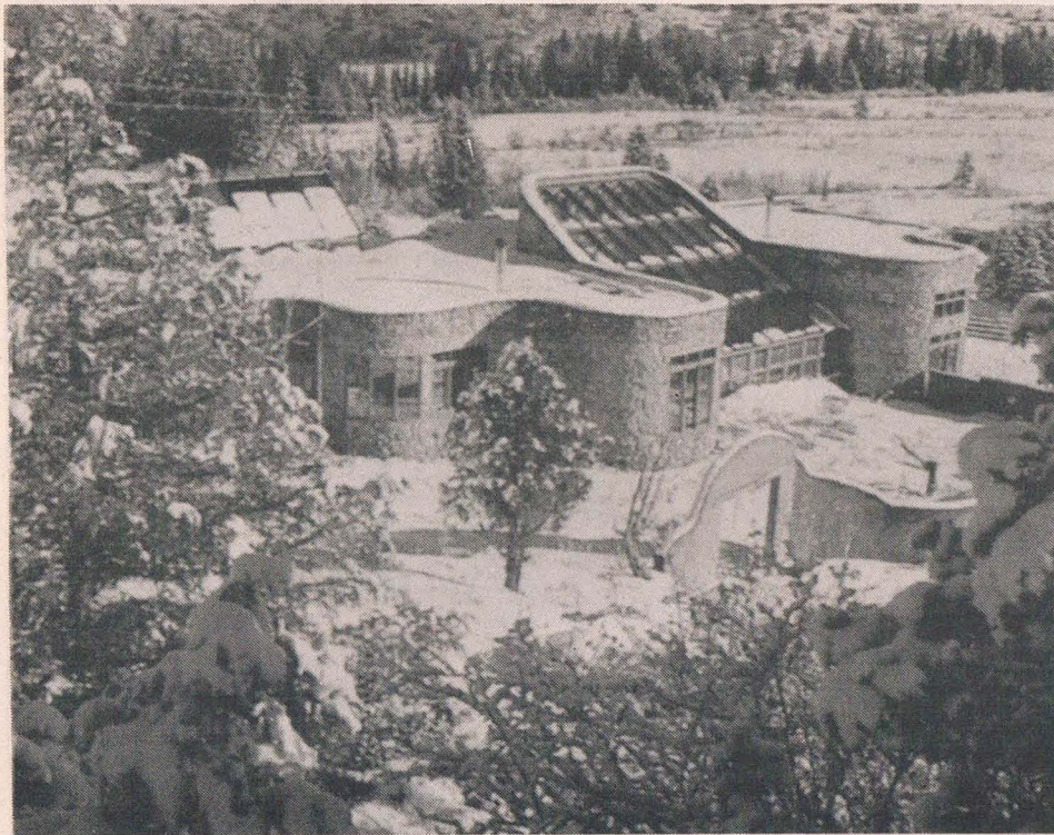
The Rocky Mountain Institute in Old Snowmass, Colorado, is a showcase of energy efficiency and includes a semi-tropical bioshelter which provides a year-round growing space for fish and crops.
