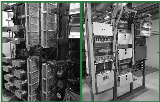
Contrasting technologies: POTS lines (left) and fiber-to-home lines (right) at Monitor Telecom in Marion County, OR, captured during a site visit by CUB Outreach Manager Sam Pastrick on August 20, 2019
